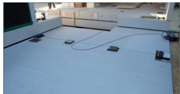
Project „Schulpavillon“, Uster/Switzerland: Vibration isolation with three different types of PURASYS vibrafoam
